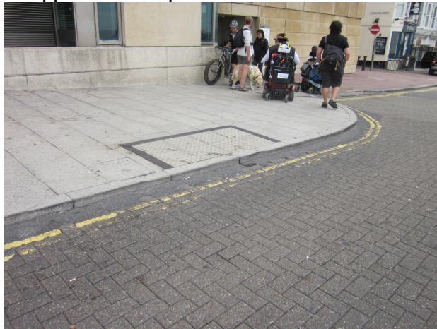
13. Kings Road near Thistle car park entrance. Tactile paving leads to a step. Dropped kerb required.
