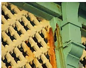
corrosion through paintwork
