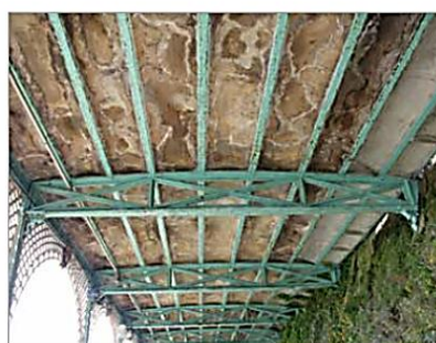
extensive weathering, cracking and spalling
