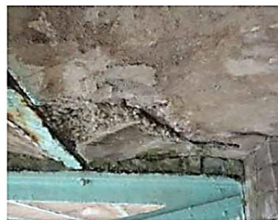
spalling, decaying jack arch
