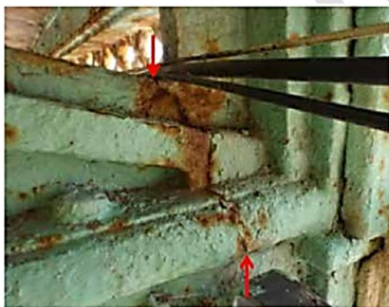
lattice beam failure
