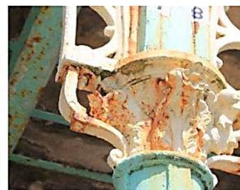
corrosion through paintwork
