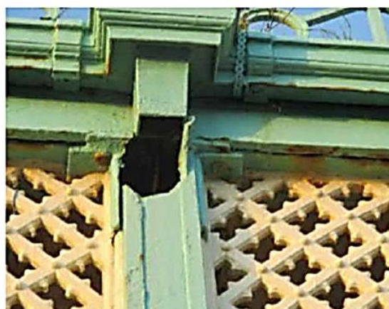
collapsed rainwater downpipe
