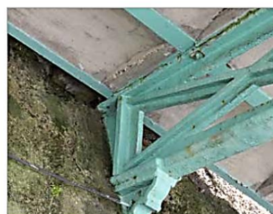
jack arch to lattice beam connection
