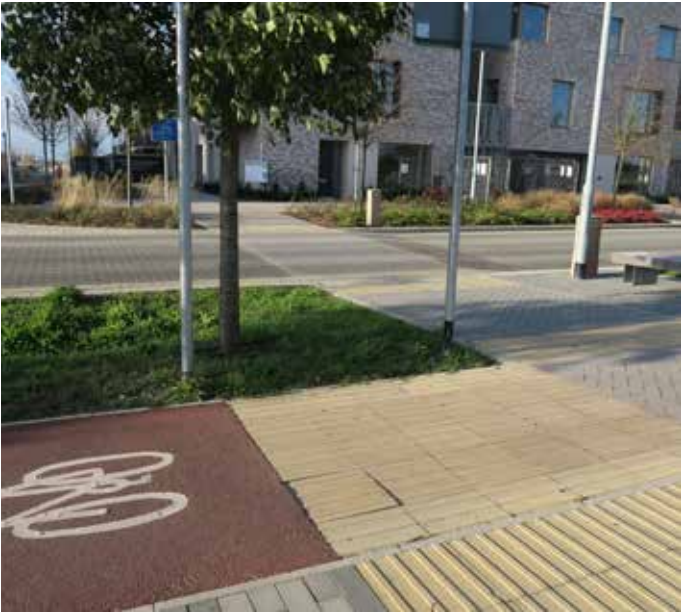
Figure 35: Example of a raised crossing across a new main road in Cambridge, with contrasting paving materials and space for low-level planting and street furniture. Note: the materials and architectural styles in this photo are indicative only; new streets and buildings in the Parish must use the materials that are appropriate to its context.
