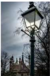
Lighting column Location: Existing light columns across the gardens Product: N/A Existing to be removed and refurbished to conservation architects detail Manufacturer: tbc Size: 6m height Colour: 'Invisible Green' (tbc)
