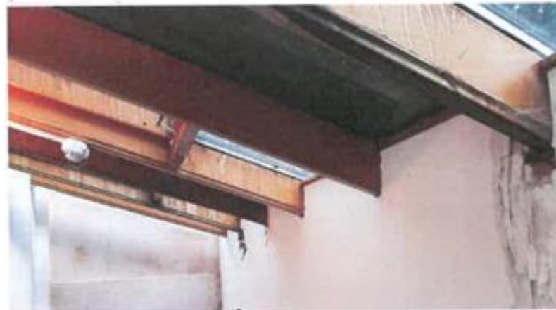
Hardwood rafters retained beneath new roof finishes
