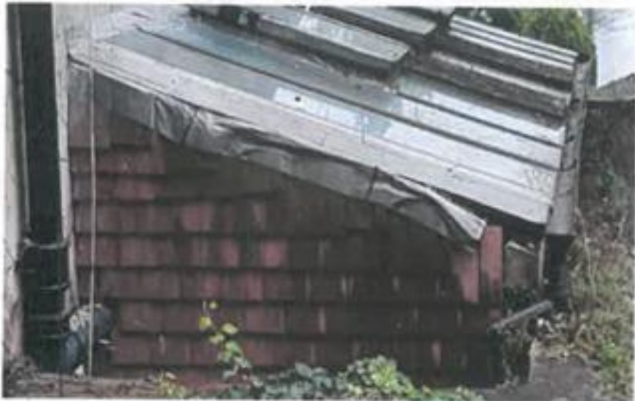
Tiles above the horizontal soil pipe connection through wall to be removed.
