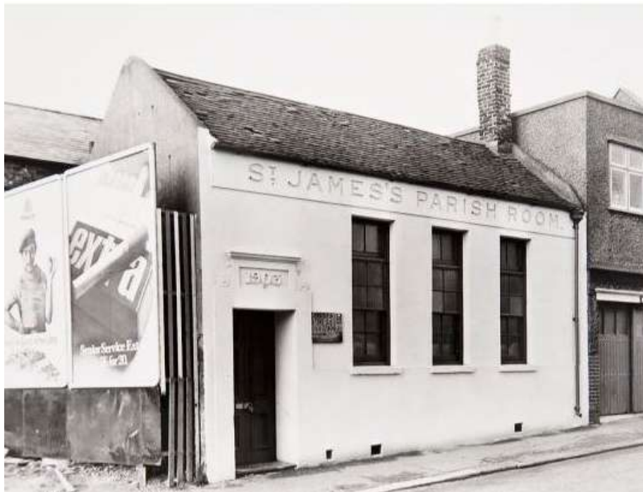
St James's Parish Rooms on High street.
