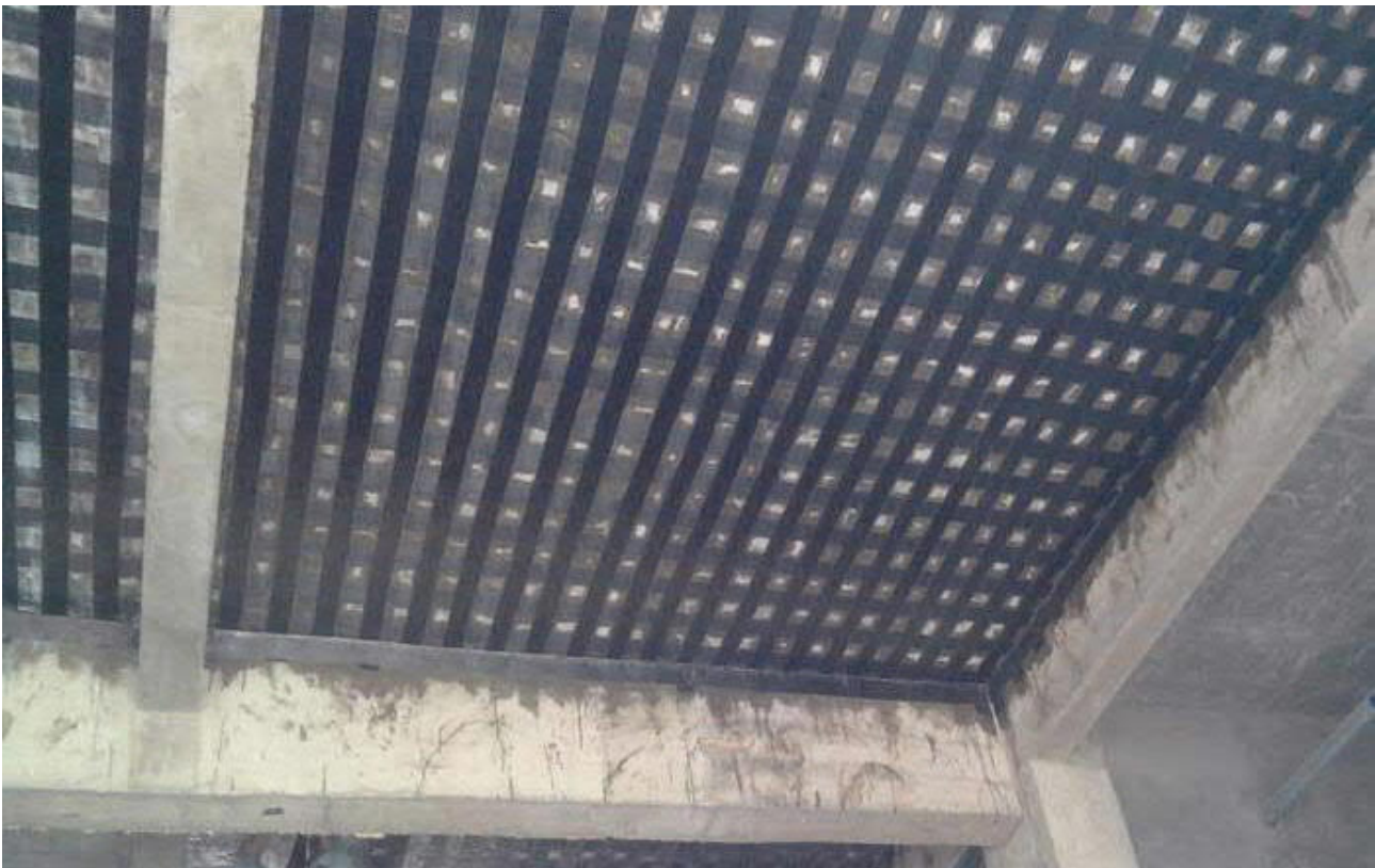
Figure 8 – Typical example of FRP strengthening
