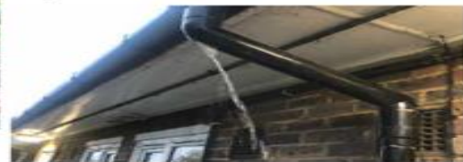
BELOW: Hollybank – overflowing gutter which was fitted only in 2017 as part of major works.
