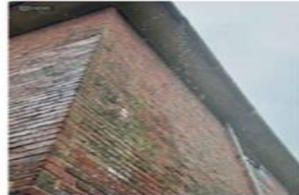
BELOW: The Cedars, taken during rainfall, showing overflow due to blocked gutter.
