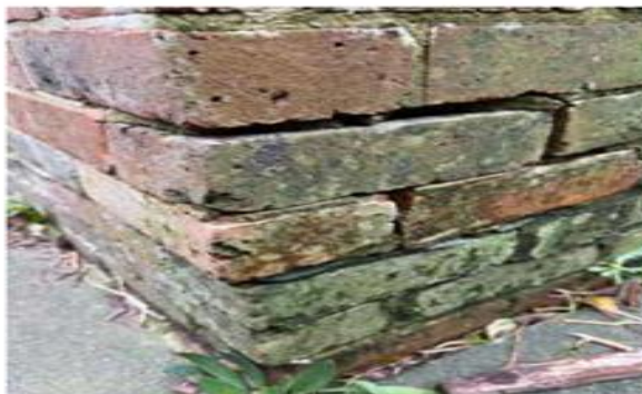
RIGHT: Hazel Bank – damage caused by broken boiler overflow, which BHCC wouldn't fix at first. Caused damp issues in three flats.
