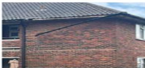
ABOVE: Guttering that has come away from downpipe and is hanging dangerously.
