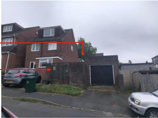
Fig 4.0 Photo of existing principle elevation, showing garage and adjacent substation.
