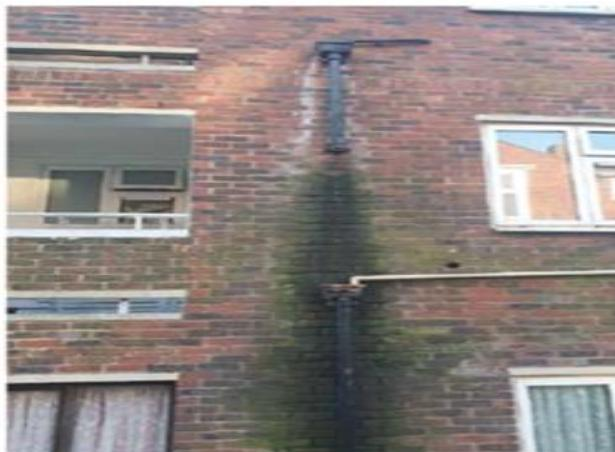
LEFT: The Lindens, showing damage caused by missing length of downpipe.
