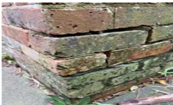
LEFT: The Cedars – loose bricks (can be almost completely pulled out) with no pointing because of exposure to rain from overflowing gutter, and causing growth of mould on internal wall. Note also the mildew on bricks.
