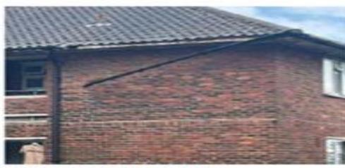
ABOVE: Guttering that has come away from downpipe and is hanging dangerously.
