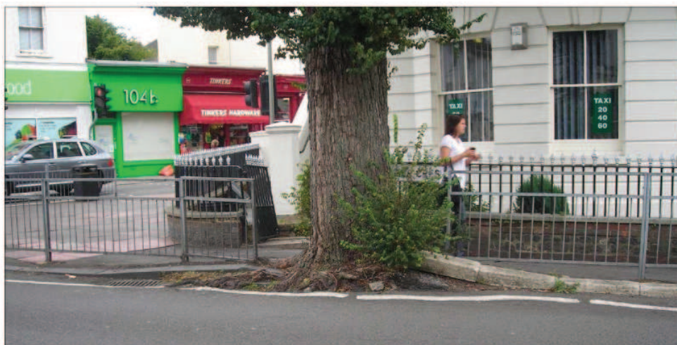
Existing carriageway and footway have been displaced / adjusted to suit the growth of the tree
