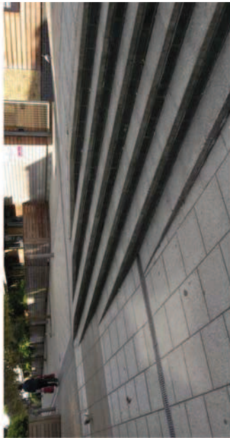
Robust material at the bottom to withstand vehicle movements and use of reflective materials at the corners to alert drivers.
