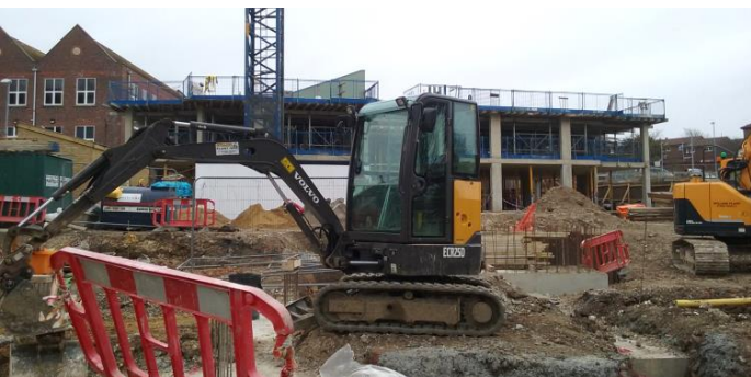
Work underway at Hobby Place
