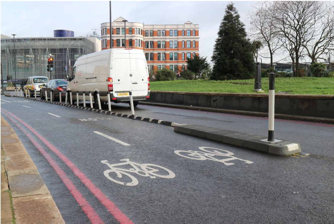
Figure 4.2: Example of light segregation (Victoria Embankment, London)
