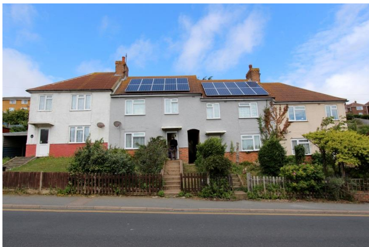
Newhaven housing stock with retrofitted PV panels (Photo: Lewes DC)
