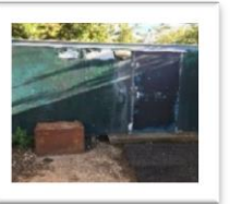
1. Greenkeepers shed 2m x 4m
