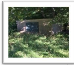
7. Storage shed 3.5m x 4m
