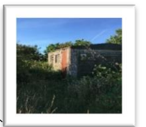
5. Pumphouse 5m x 3m
