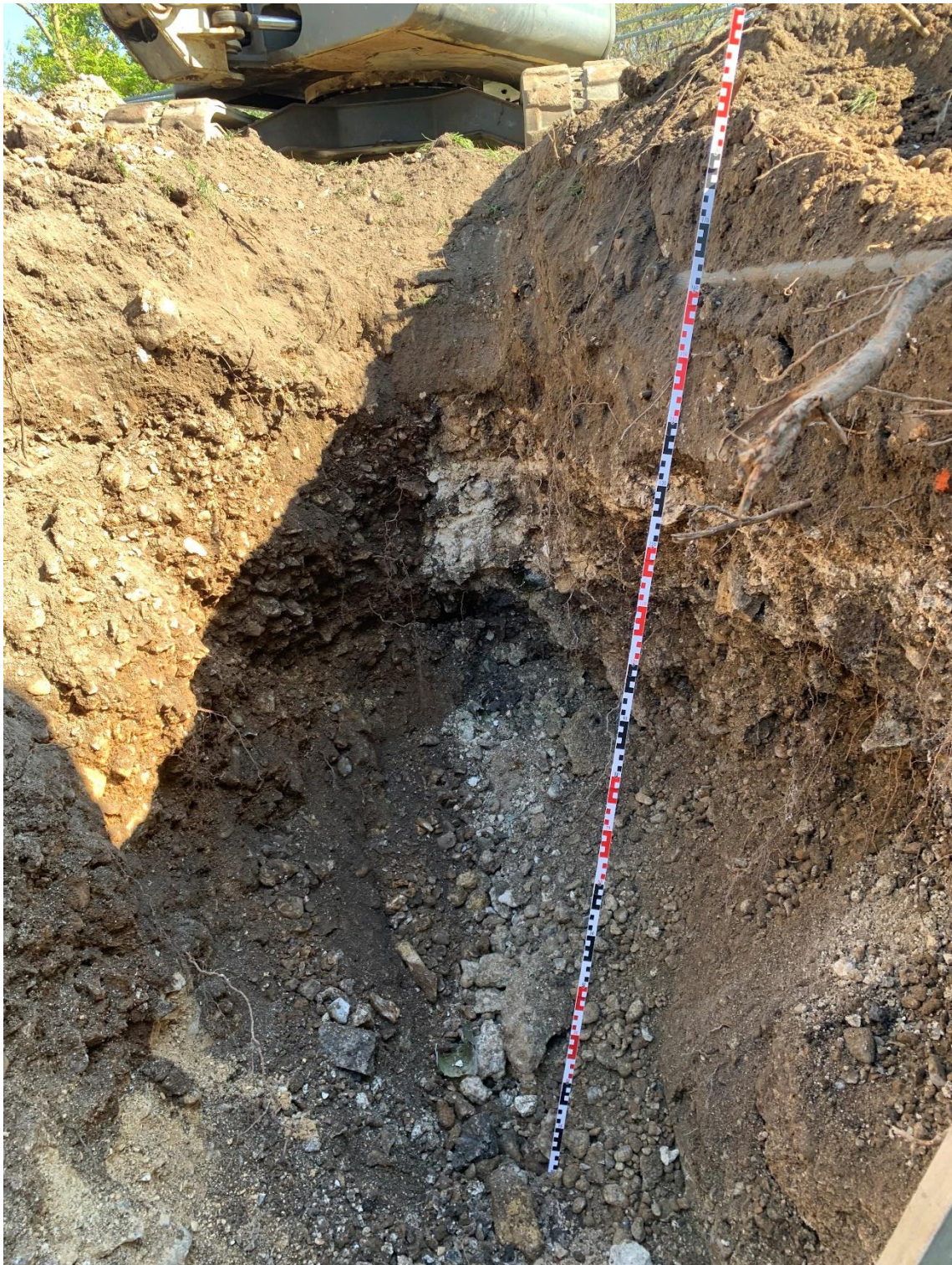
Photograph 6: Trial hole excavated 27 April 2022 (looking north) showing filled nature of ground and chalk filling on the side of the nearby sewer.
