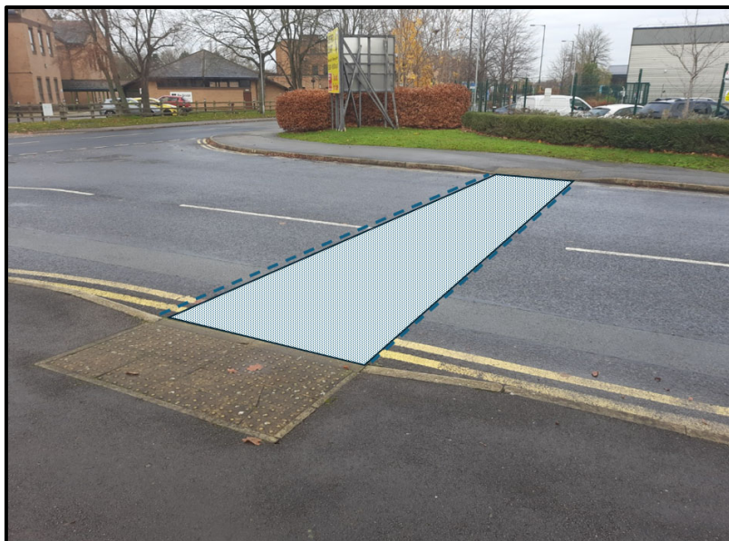
Designated tactile crossing point – adjacent to road junction
