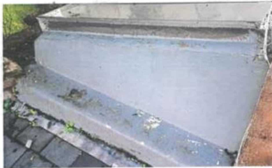
Rendered finish to be overclad with leadwork
