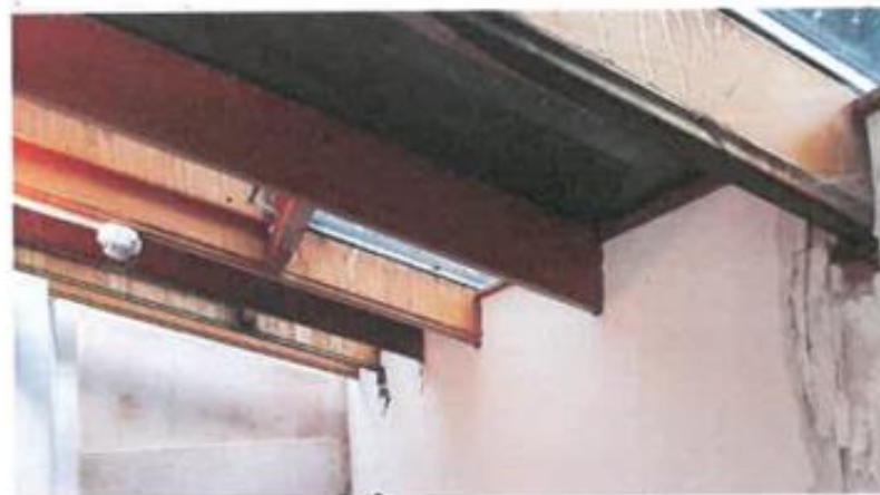
Hardwood rafters retained beneath new roof finishes
