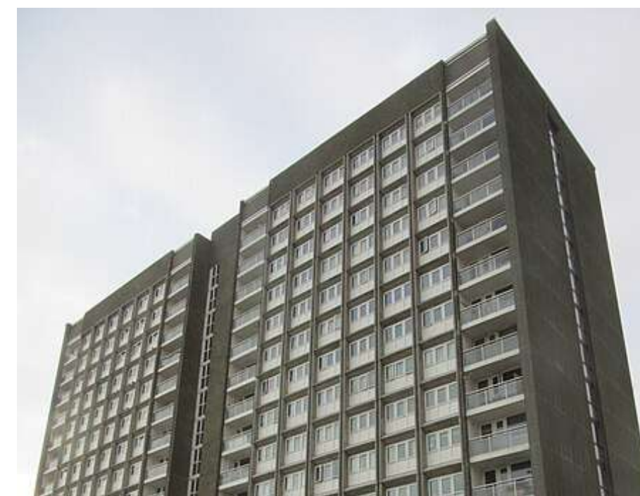
St James's House - current apperance, subject to structural review and possible demolition .
