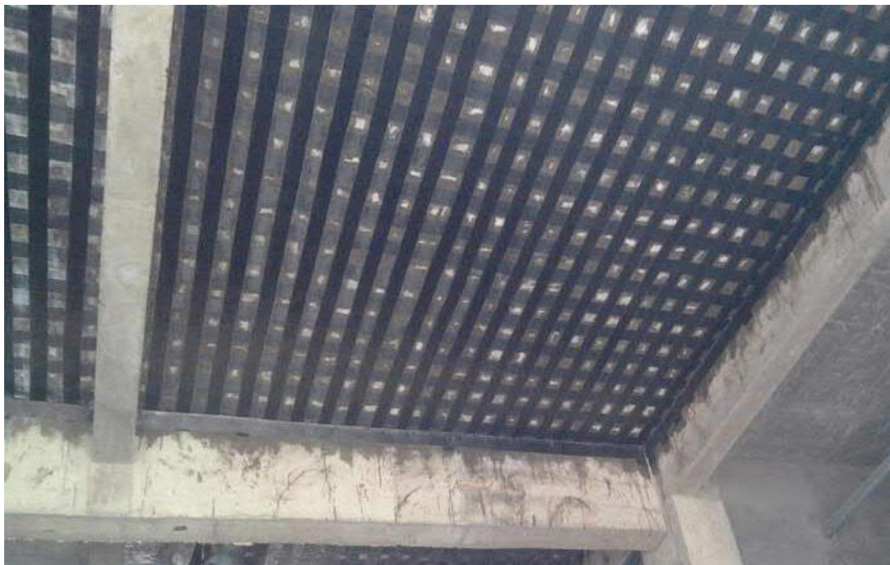
Figure 8 – Typical example of FRP strengthening
