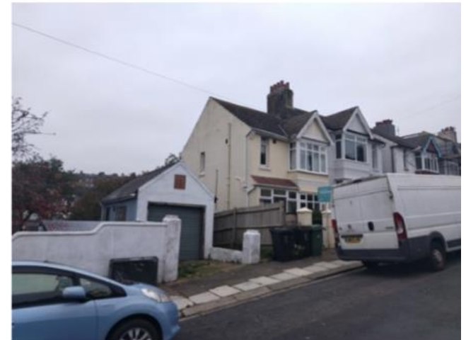
Fig 4.5 Photo of No.165 Hollingdean Terrace.
