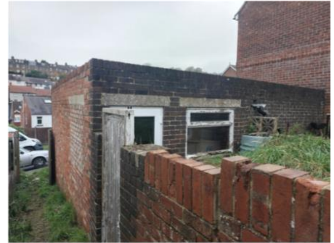
Fig 4.2 Photo of existing garage entrance and retaining garden wall.
