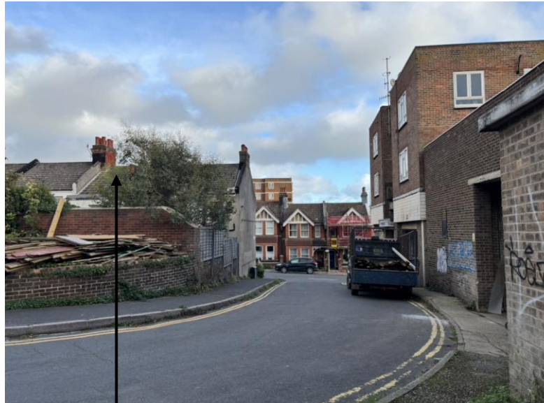
Rear of properties on Tillstone Street
