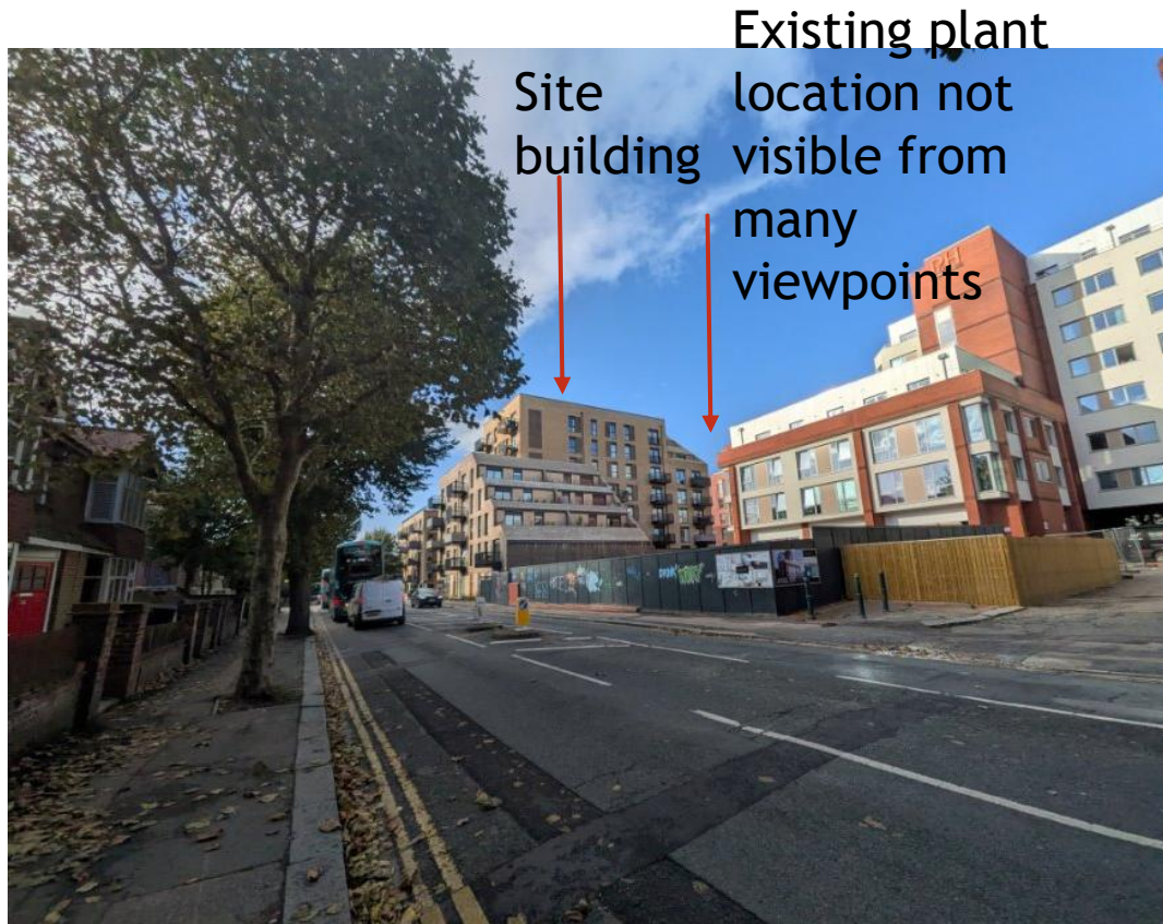
Looking West along Davigdor Road - East elevation of site with the existing plant not visible
