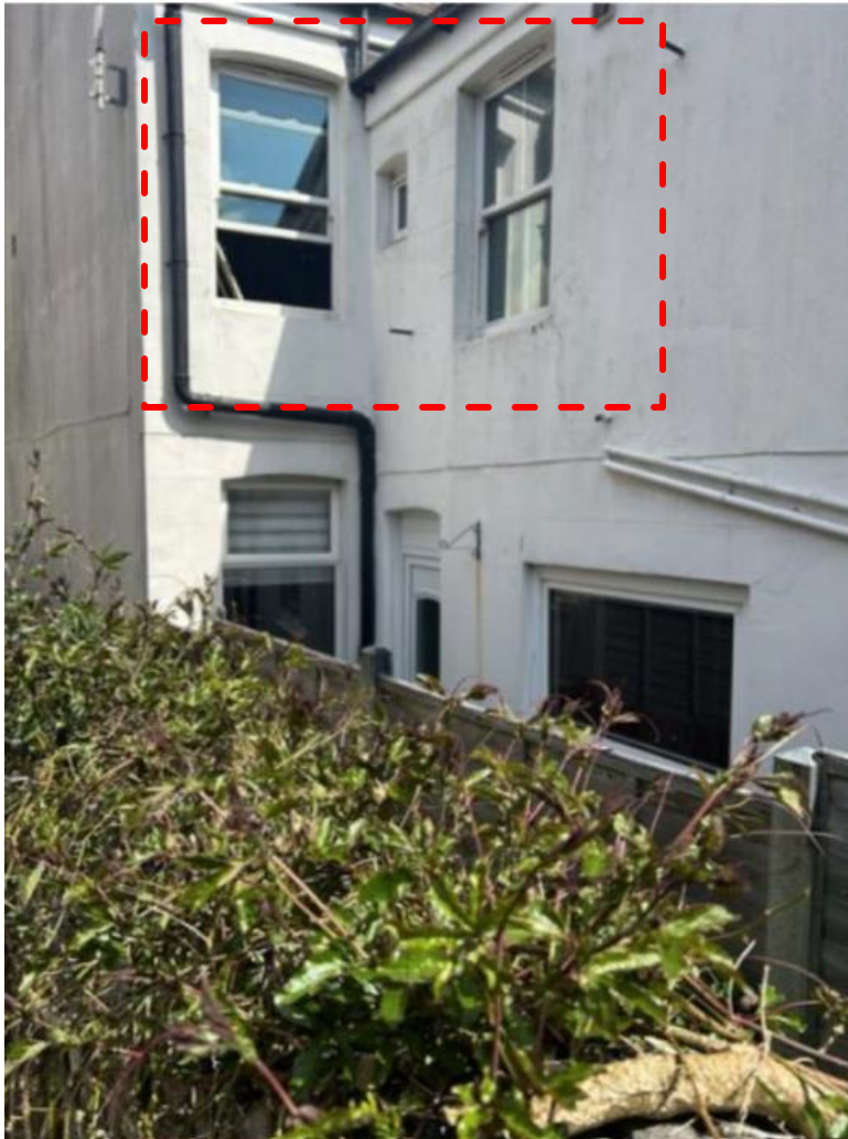
Windows on No 35 on West elevation
