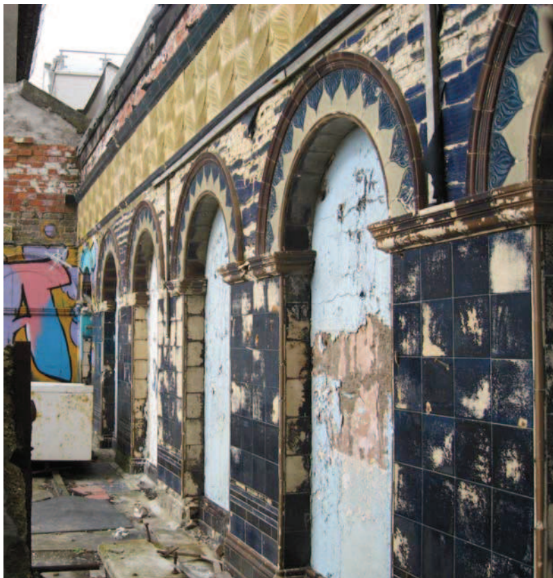
Original ceramic tiles attached to the north east wall of the former swimming baths, Medina House site, Kings Esplanade
